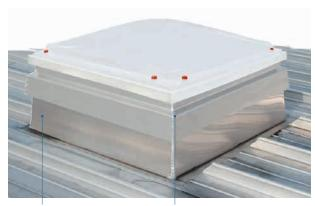
Aluminium outer shell welded to the roof covering
